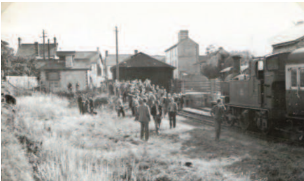
Figure 2. Cowbridge railway station 13
